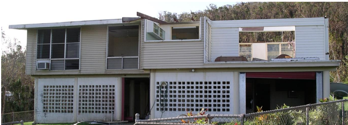
Figure 16. Roofing and wall damage to a high-set 1970s home as presented to builders, assessors, and engineers for experience based estimates of repair cost
